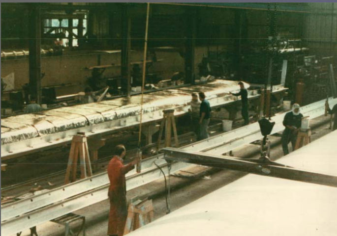
Roof assembly under construction.
